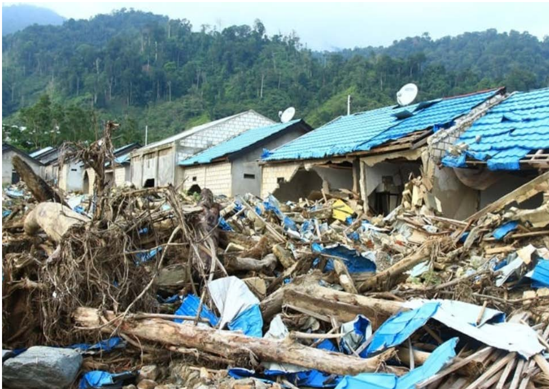
Figure 3 Settlement Damaged by Flash Flood in Sereh Village
